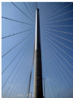
Figure 2: Mono tower and stay cables
