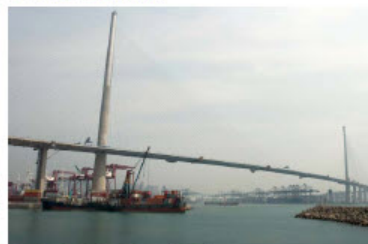
Figure 1: General view of Stonecutters Bridge
