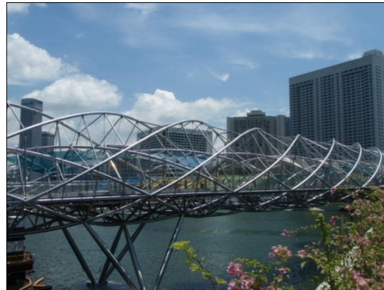
Helix Bridge, Singapore, 2011
